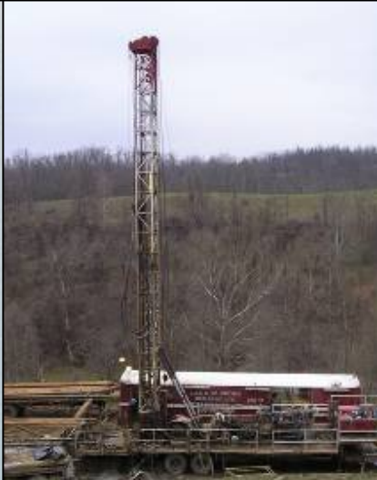
Regional Reservoir Characterization “Piggyback Drilling”
